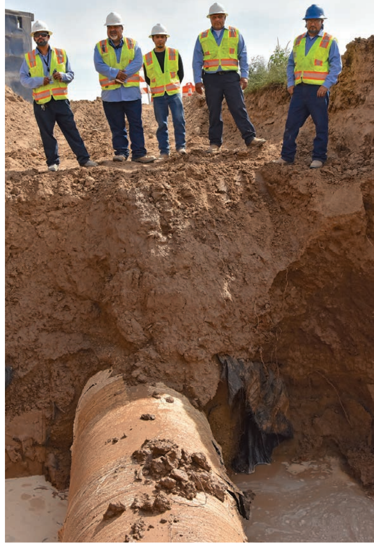
El Paso Water team members Norman Escarcega, Norberto Olmos, Bryan Sanchez, Armando Gonzalez and Norman Escarcega (from left) on site to repair a 48-inch water main break.
