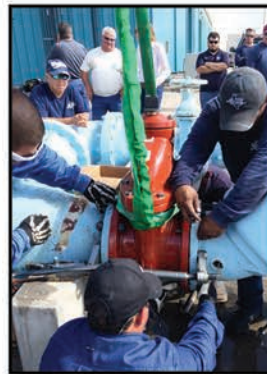
Reinstall new valve
