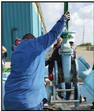
Spread outside flanges & remove old valve
