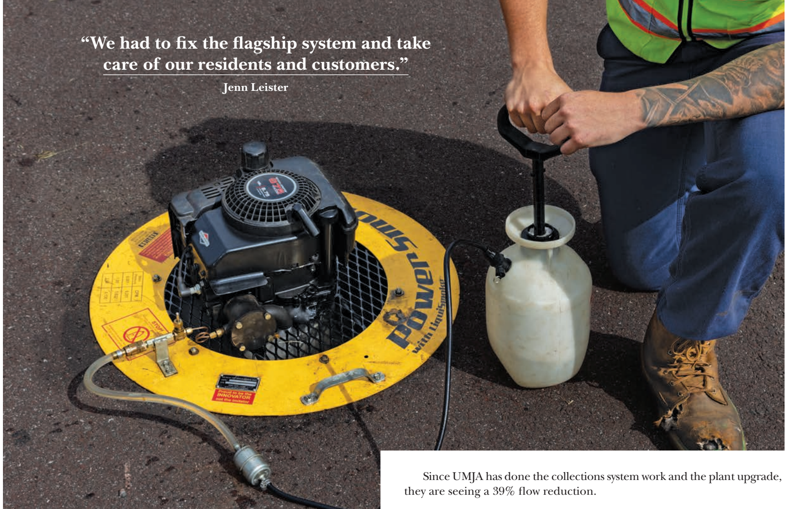
A crew member uses a Hurco Power Smoker to identify sewer system inflow and infiltration points.
