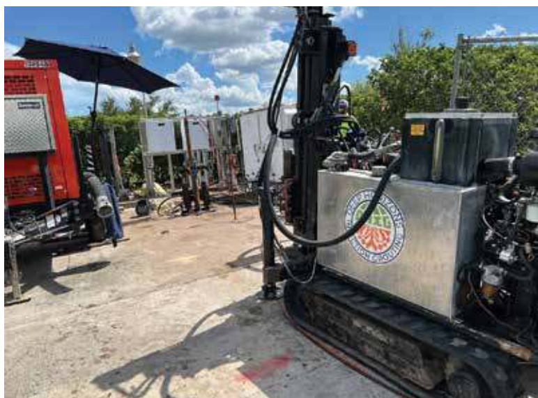
The small equipment footprint allows easy access in tight spaces. The five-day project included four injection points and 2,623 gallons of grout.
