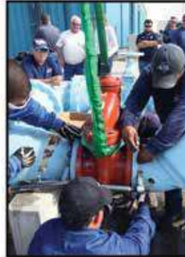
Reinstall new valve
