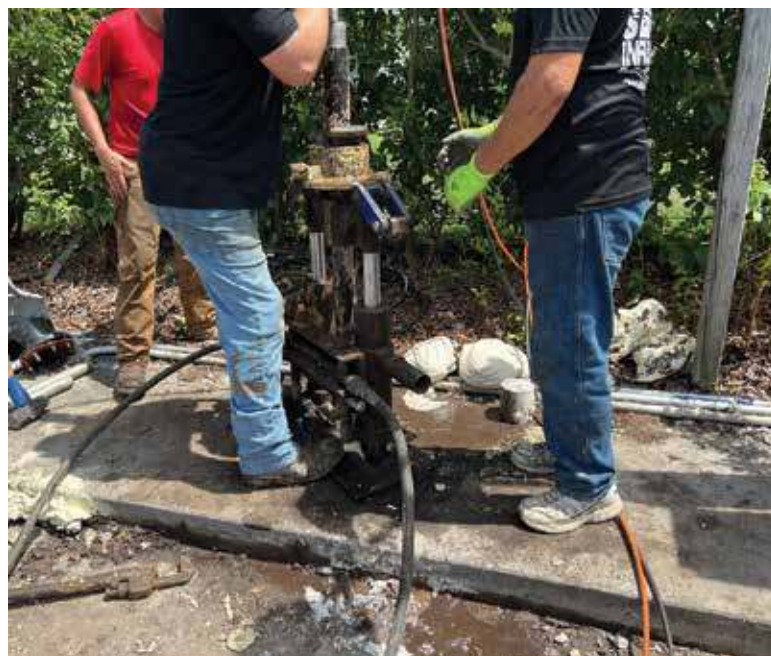
A crew deploys the patented mixing device to 31 feet adjacent to the 10-foot void near the wet well.
