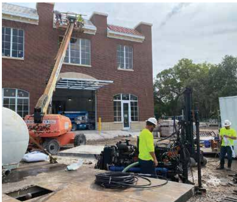
Installers inject dual-component polymers to seal Sarasota Lift Station 87 while construction continues.
