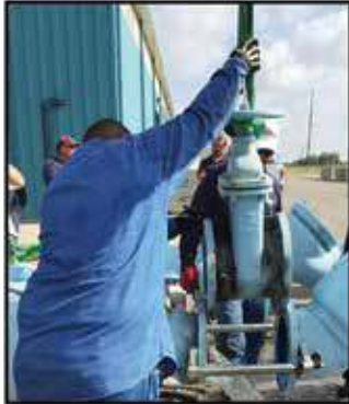
Spread outside flanges & remove old valve
