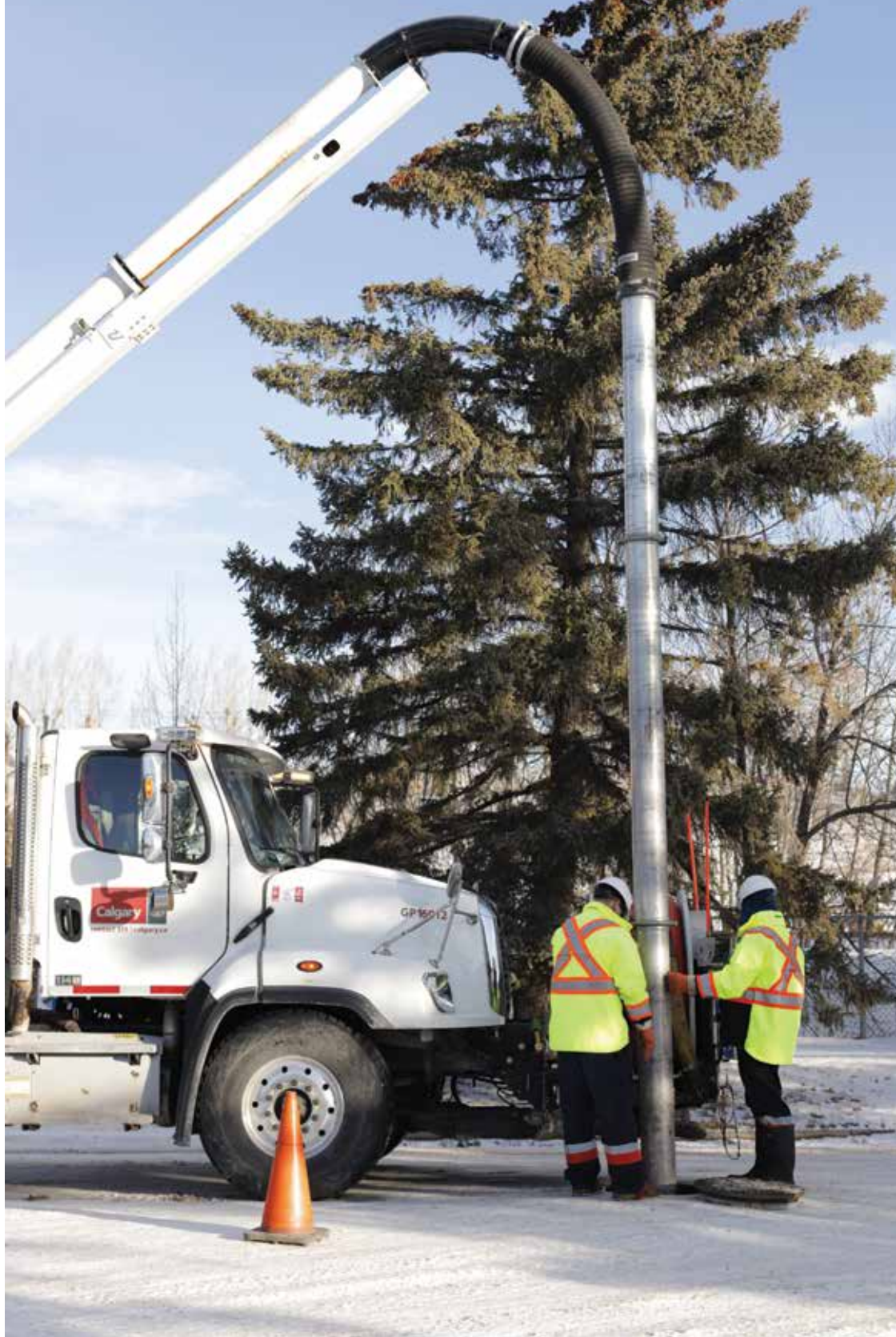
Moore and Aman Sran vacuum debris from a manhole with a Vactor 2000 jet/vac truck.
