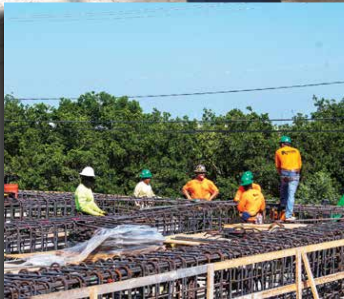
Left: Crew members lay rebar for the FKAA's new generator building. Each piling is more than 3 feet in diameter to anchor the foundation in place if a catastrophic hurricane hits.
