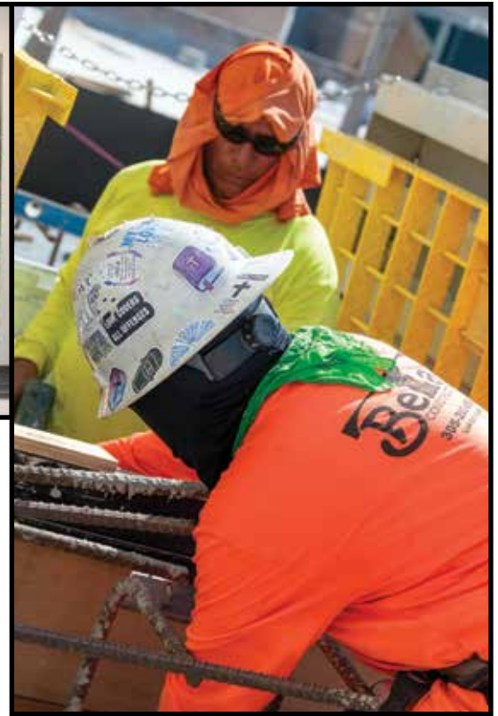
Construction of the FCAA's new desalinization plant on Stock Island is scheduled for completion within the next two years.
