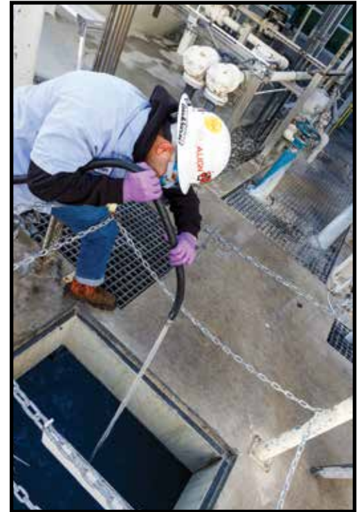
Rodrigo Ibarra works on pigging the lines at the GWRS plant.
