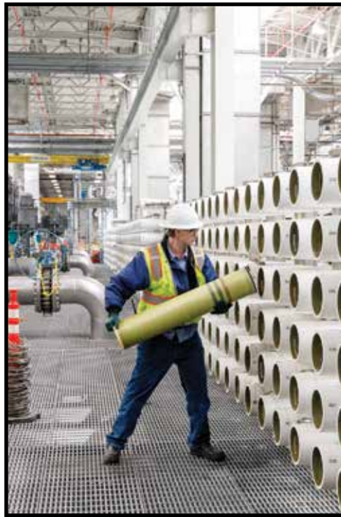
Mike Ewing performs a reverse osmosis membrane change using LD Technology's ESPA2-LD.
