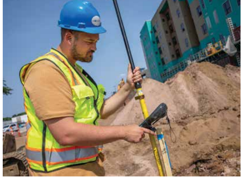
An inspector from Infrastructure Design Group takes measurements at the job site with a Trimble R8.
