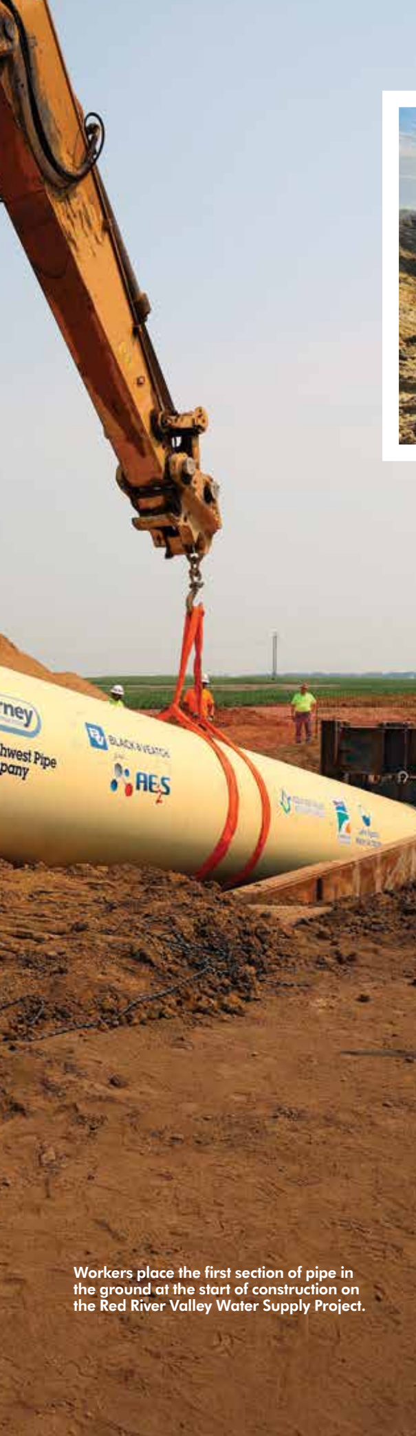
A crew installs a corner section of pipe east of Carrington, North Dakota.
