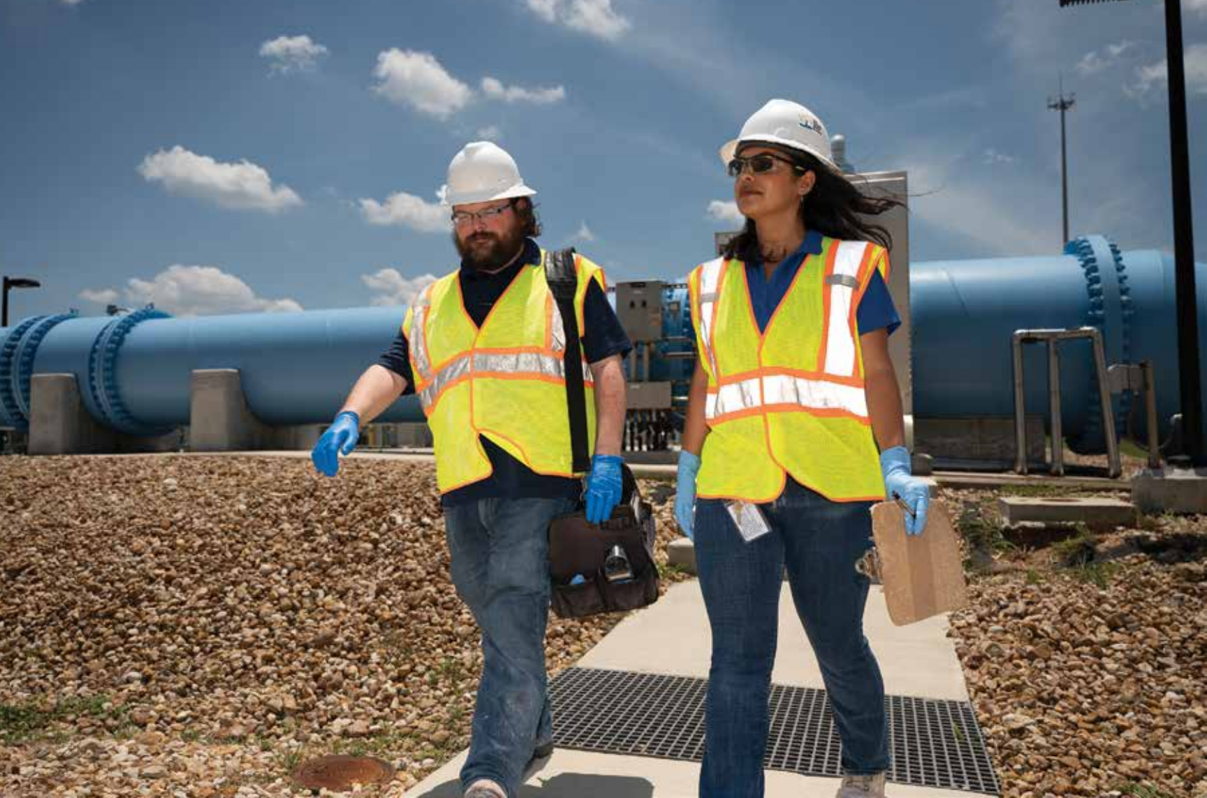
Nolan Paige and Krystal Accuosti are operators at San Antonio Water System's Aqua Vista Plant in North San Antonio, which conditions water brought in from the new 142-mile-long pipeline.
