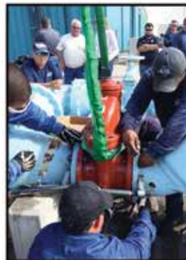
Reinstall new valve
