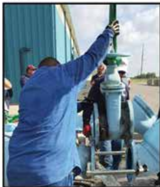
Spread outside flanges & remove old valve
