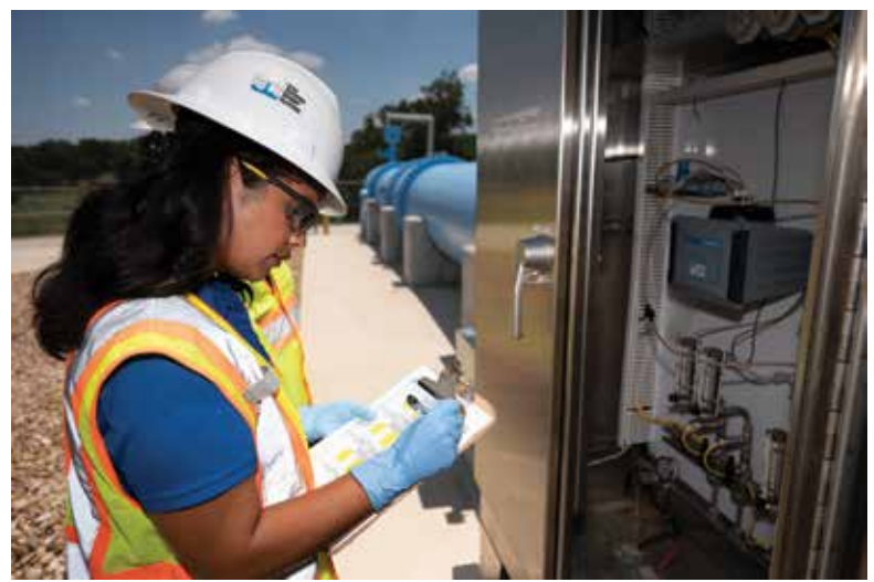
Krystal Accuosti checks equipment readings at the Aqua Vista Plant.
