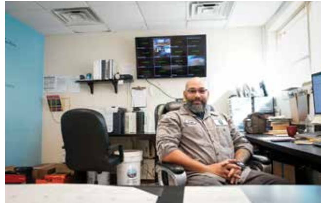
Ángel Negrón Monllor is the lead operator at the Northeast Wastewater Treatment Plant.
