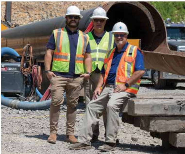
Water Production Manager Cody Howell, Project Manager Todd Piller and Utilities Director Monty Ledbetter (from left) at the exit point of the 2,600-foot tunnel that will bring freshwater from Lake Ouachita through Blakely Mountain.
