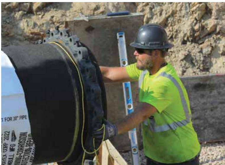
Work continues on Hot Springs' new water treatment facility.
