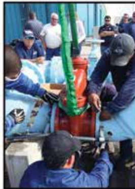
Reinstall new valve
