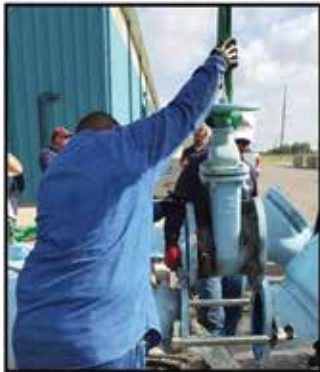
Spread outside flanges & remove old valve
