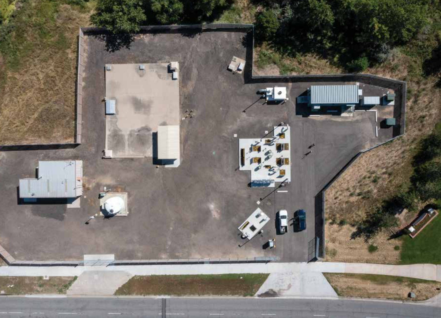
The 4.5 mgd lift station collects nearly all of Northglenn's sewage and pumps it 11 miles through a 27-inch force main to the wastewater treatment plant.
