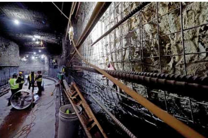
Concrete forms line the walls and ceiling of the tunnel.
