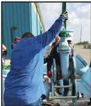
Spread outside flanges & remove old valve
