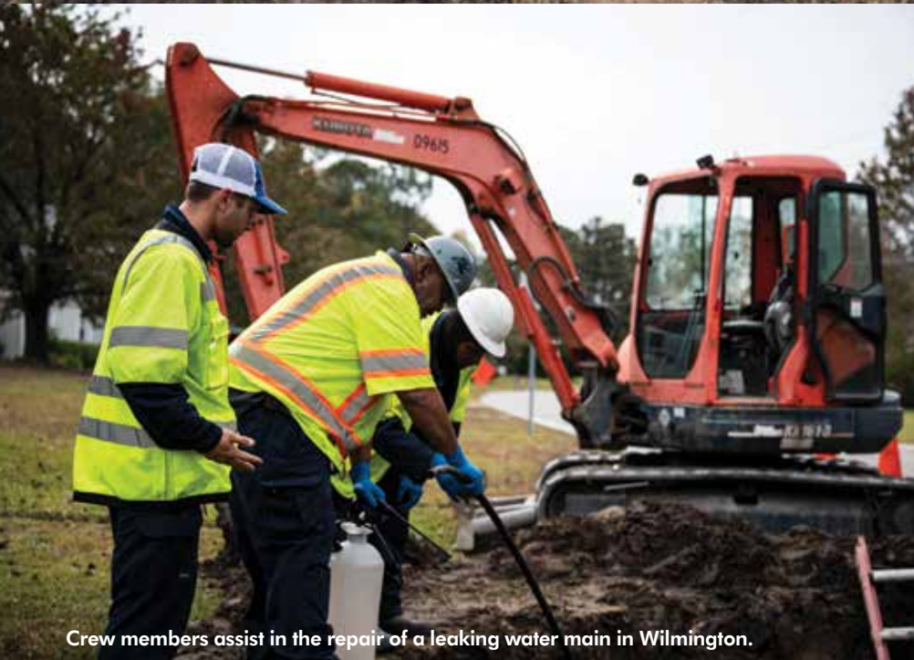
Crew members replace a damaged section of water main with a new piece of PVC and Macro couplings from Romac Industries.
