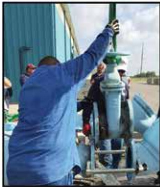
Spread outside flanges & remove old valve
