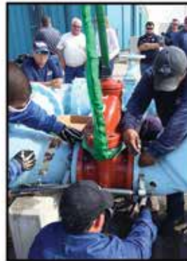
Reinstall new valve
