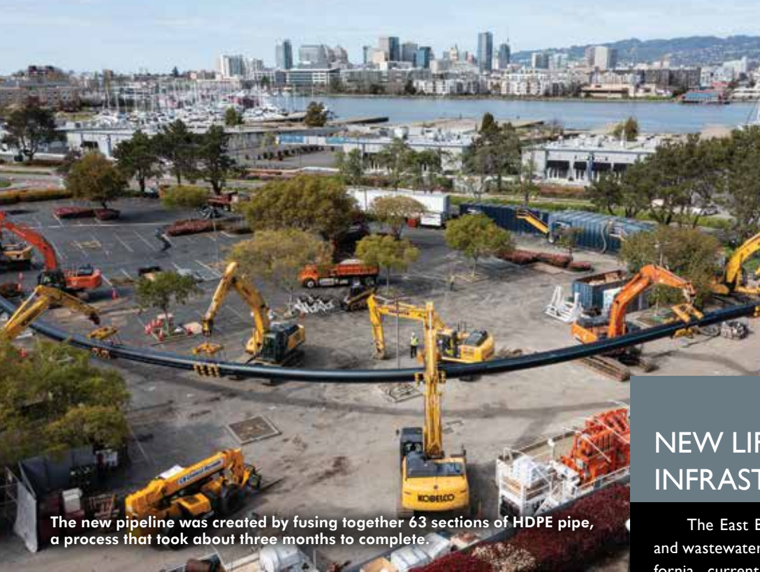
Construction began in summer of 2022. About half of the bore was drilled from the Oakland side of the harbor and the other half from the Alameda side.
