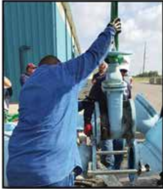
Spread outside flanges & remove old valve
