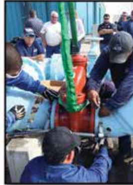
Reinstall new valve
